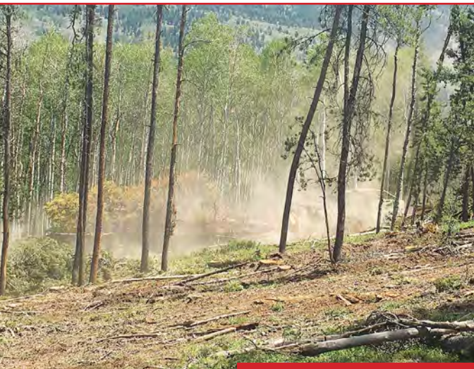
Skidding operations exposing bare mineral soil. Photo: CSFS
