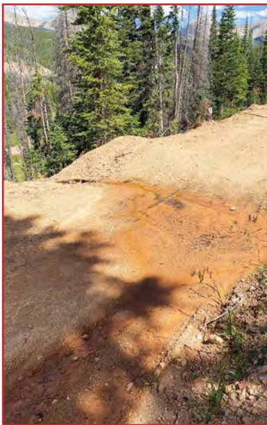
Waterbar diverting surface drainage and reducing velocity of runoff. Photo: CSFS
