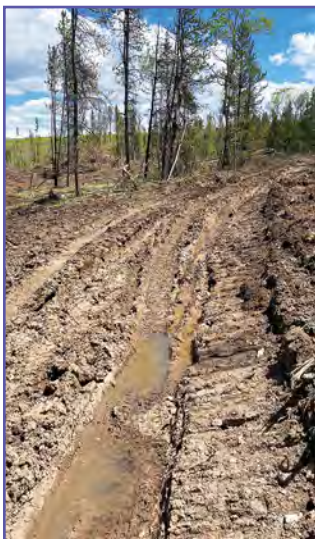
Temporary road constructed through ephemeral draw. Photo: CSFS
